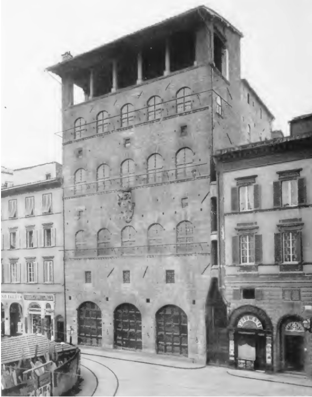
Figure 4. Palazzo Davanzati, Florence, showing a nearly the full menu of façade possibilities with loggia, rustication at street level, rough stone above, and a virtual advent calendar of windows for public display. 30
